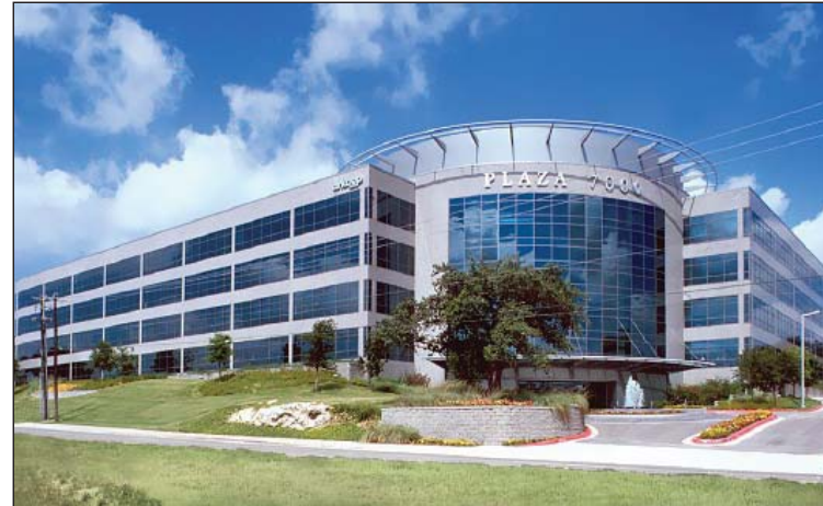
Nirvana Systems Inc. Headquarters in Austin, Texas.
